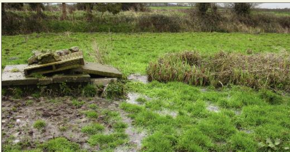
A malfunctioning domestic wastewater treatment system photographed by Anne Goggins of Limerick County Council is typical of thousands of such systems across Ireland. As Paul Hynds and Owen Naughton discovered, lack of information and awareness are significant contributors to such problems.
