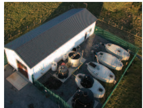
Milltown WTP, Co. Galway
