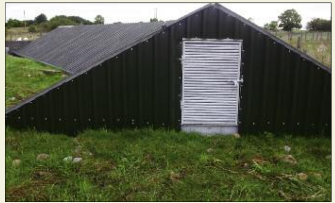
Killaturley GWS well-head has been covered as part of a major upgrade. A sluice gate has been positioned at the outflow from the well-head site to ensure that there is a sufficient raw water supply in periods of drought.
