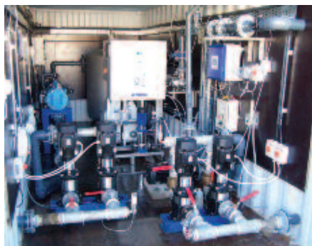
Burrishoole Temporary WTP, Co. Mayo
