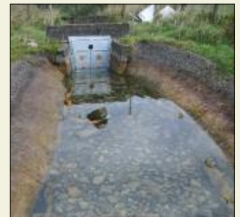
Killaturley GWS well-head has been covered as part of a major upgrade. A sluice gate has been positioned at the outflow from the well-head site to ensure that there is a sufficient raw water supply in periods of drought.
