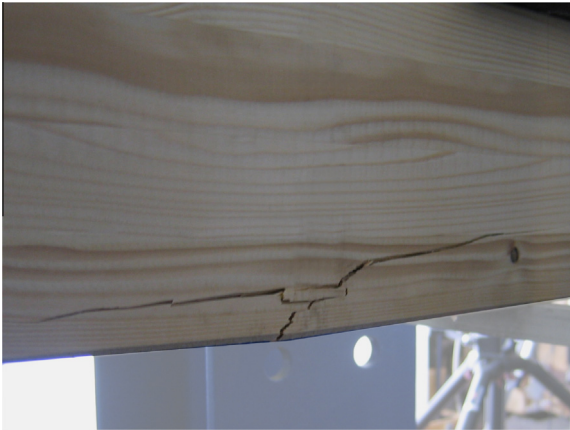
Fig. 7. Tension failure under bending.
