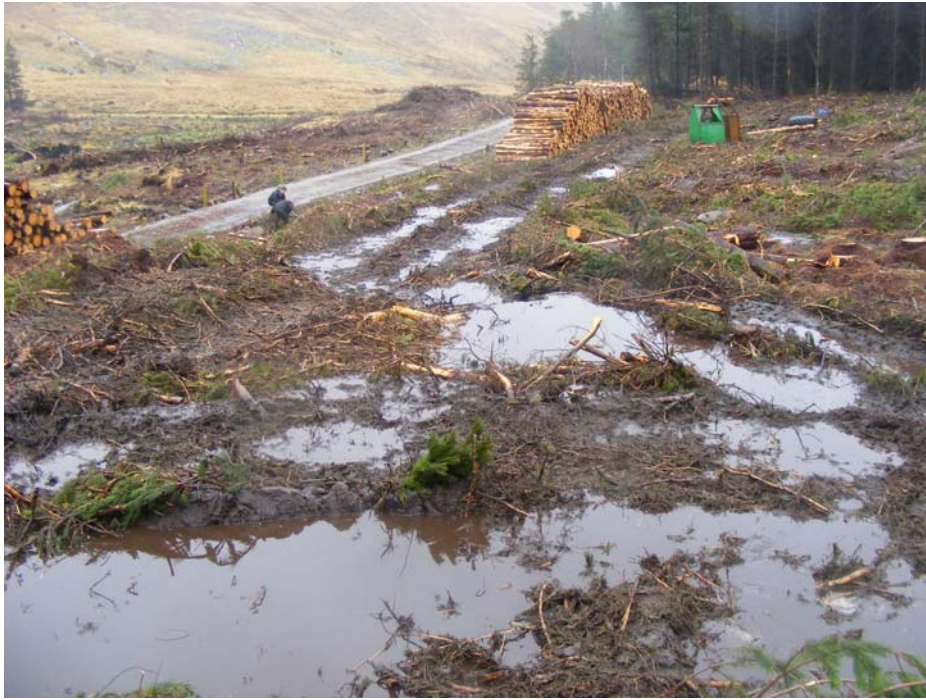
Figure 6.4 Ponding of water following heavy rainfall during clearfelling.
